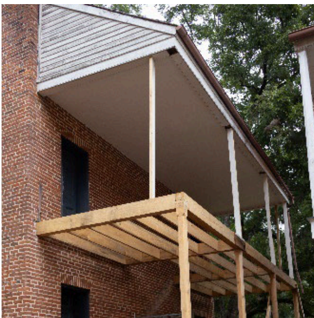
Construction of the steward's porch.
