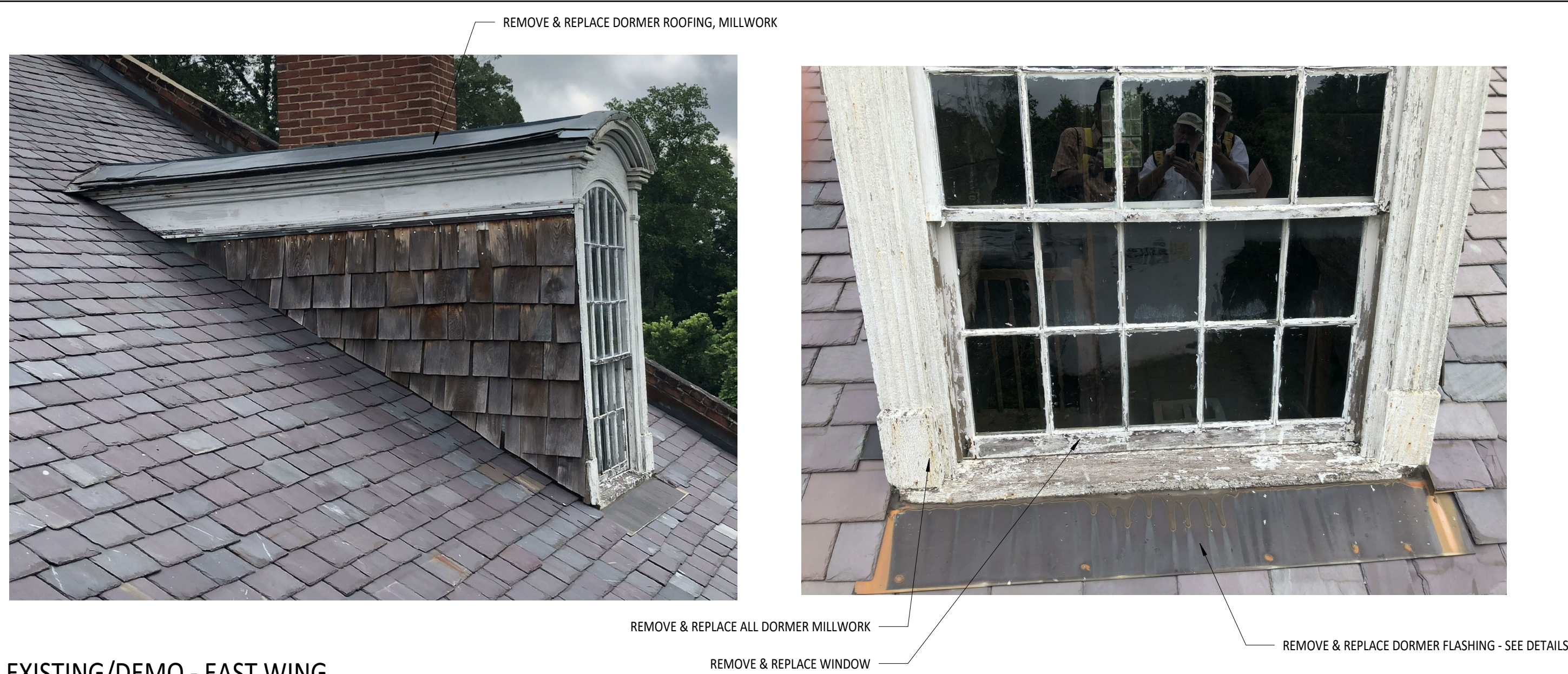
EXISTING/DEMO - EAST WING
