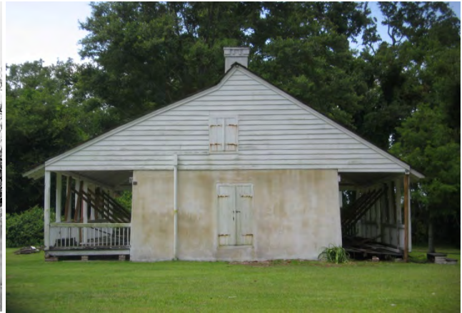
Figure 6-2. East side of La Pointe-Krebs House in 2010.
