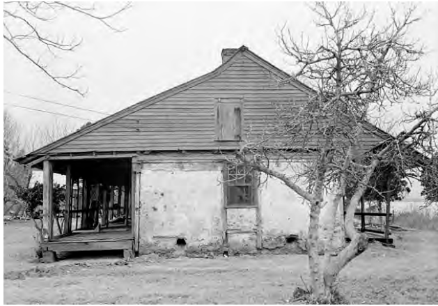
Figure 6-1. East side of La Pointe-Krebs House in 1936 (Historic American Buildings Survey, National Park Service).
