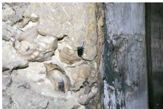
Figure 6-10. Detail of a tabby in-filled wall of the east room of La Pointe-Krebs House, prior to the 1995 restoration.
