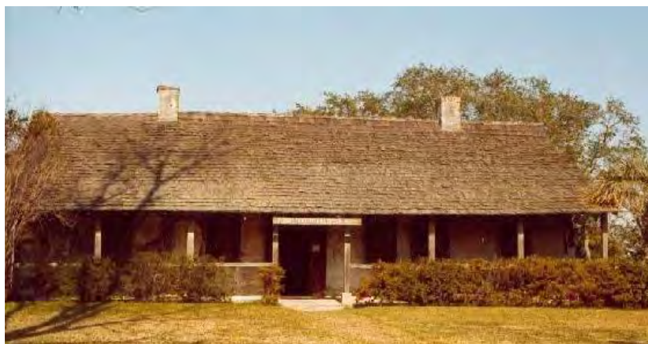
Figure 2-42. Undated photograph of the south side of La Pointe-Krebs House with row of bushes that were pulled out prior to the 1995 restoration, damaging archaeological deposits in the process.
