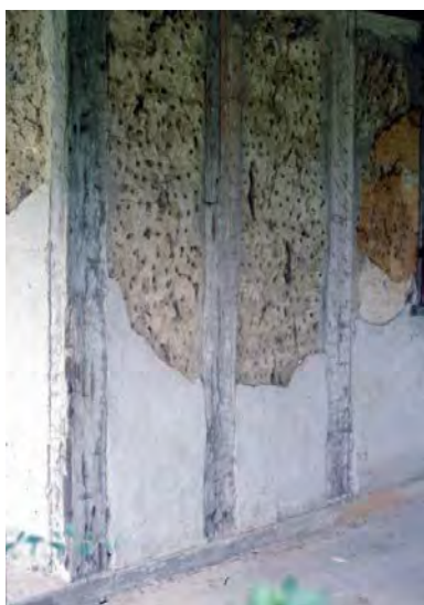
Figure 6-9. Detail of a plaster-covered bousillage in-filled wall of the west room of La Pointe-Krebs House, prior to the 1995 restoration.
