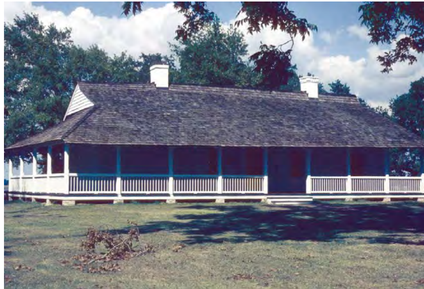
Figure 1-14. La Pointe-Krebs House after the 1995 restoration.
