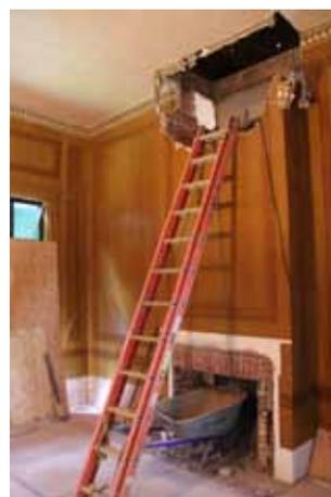
used to carefully raise the lower sections to the level of the highest corner. To minimize damage to the plaster walls the sections will be moved no more than 5/8" each day.
