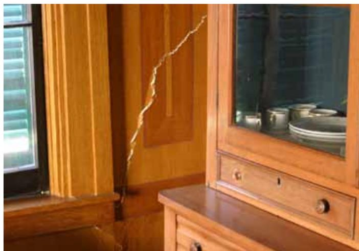
A crack in the plaster wall of the dining room that has ripped through the hand-grained faux wood finish wallpaper.
