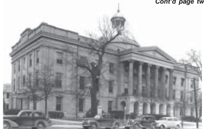
The Old Capitol, late 1930s, its exterior covered with stucco colored and scored to replicate limestone.
